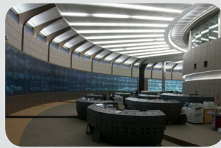
Railway control Center
